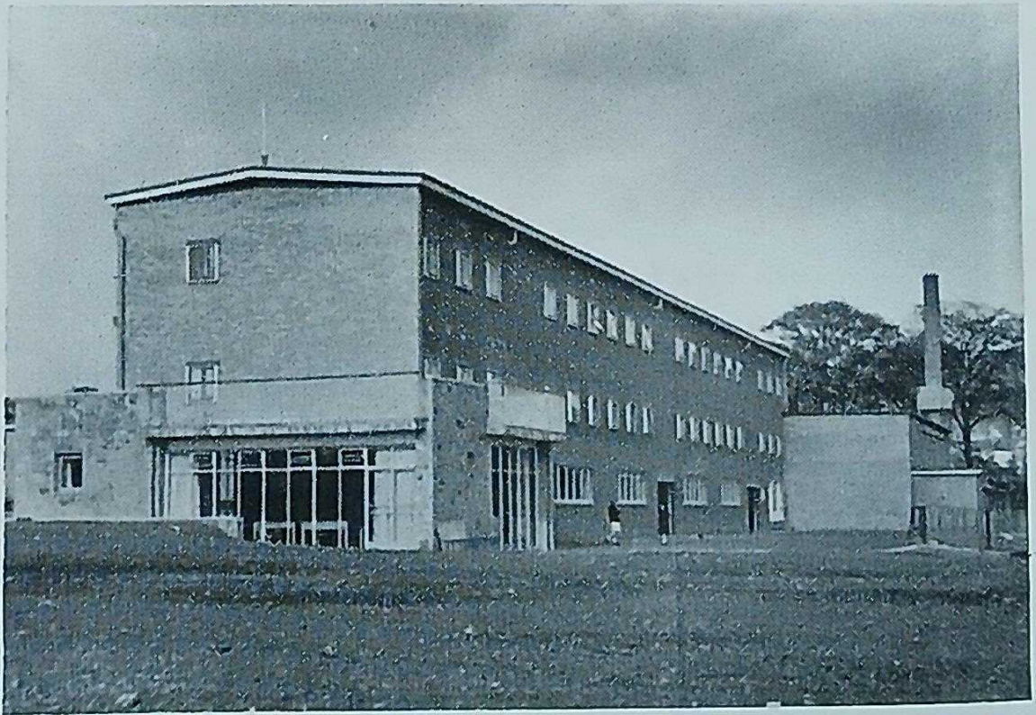
THE NEW SCHOOL, DUDDINGSTON ROAD
